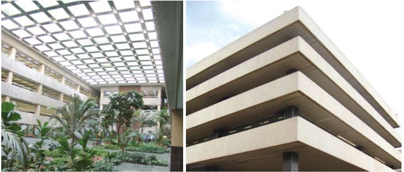
SARS Large Business Office at Megawatt Park
